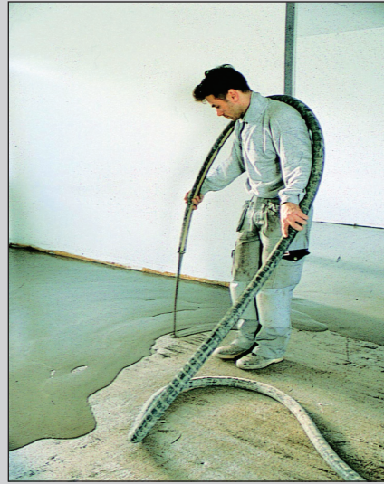
Warehouse with ABS 410 floor for wear resistance
