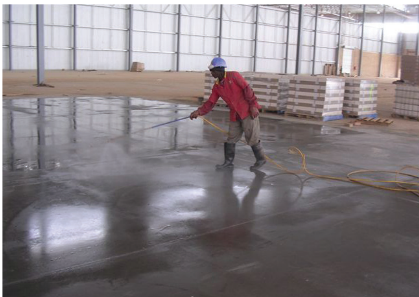
Spraying on CLF Super Seal
