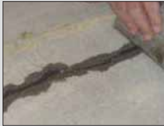
6. Excess material is trowelled or scraped off before curing.
