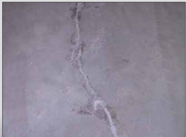
Crack after repair
