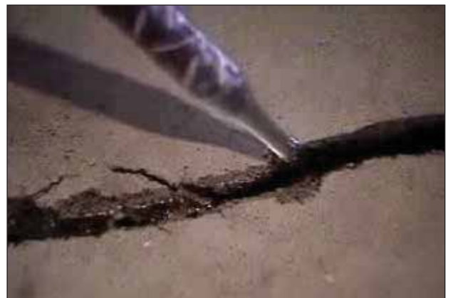
Saturate the Crack with Roadware
