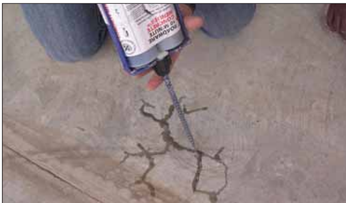
Repair of Surface Delamination
