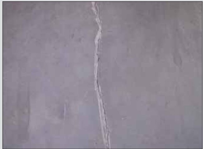
Crack prepared and ready for treatment
